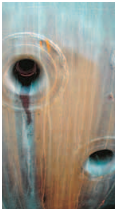
HMS Gotland's discharge pipe. Modification of the submarine included the replacement of drainpipes to a quality that withstands warm, salt water. Parts of the seawater bearing system are, however, still adapted to the colder waters of the Baltic Sea. That is why vents, pipes and pumps are thoroughly checked.
